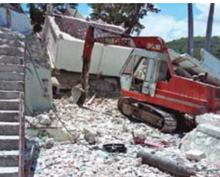
Out of the rubble, our new facilities emerge.
